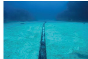
[ Cables laid on sand to avoid coral reefs ] [ Debris collected from the seabed ]
