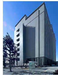
[ Saitama 1 Data Center (100% powered by renewable energy from fiscal 2022) ]
